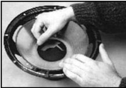
**Step 5 – remove the dust cap from the middle of the cone**
